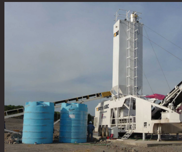
Dam building Mexico
