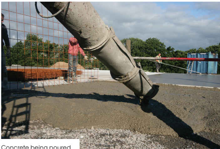
Concrete being poured
